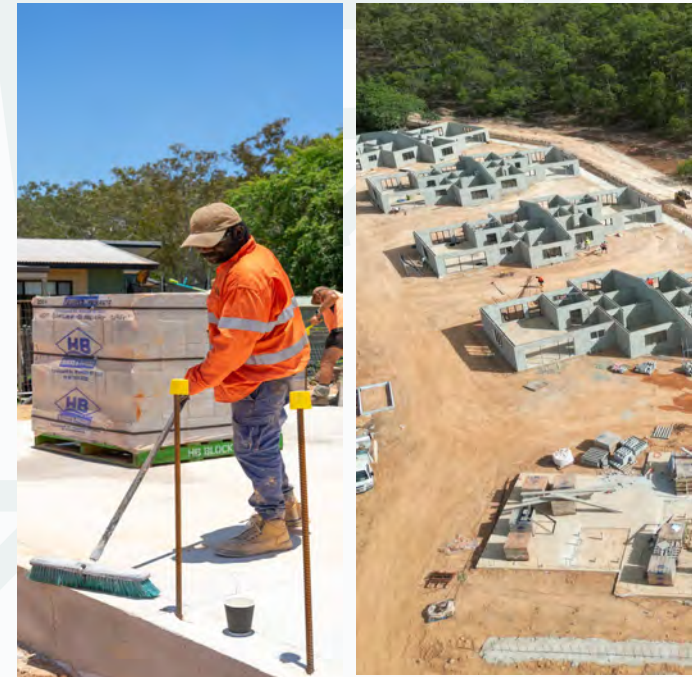
Rirratjingu Housing Development at Bunggulwuy Close
